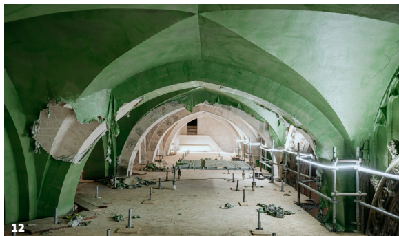
12. Cleaning of the aisle vault with latex, 25 April 2024 © City of Chalon
